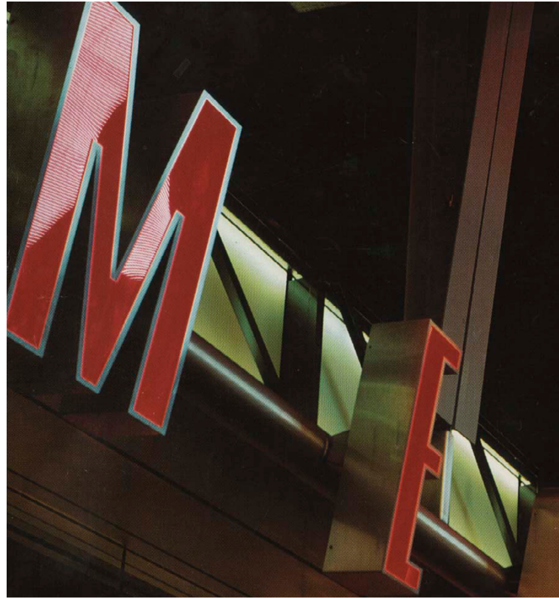
Primary Sign: Signage tube with internally illuminated metal pan letterforms and acrylic face.
