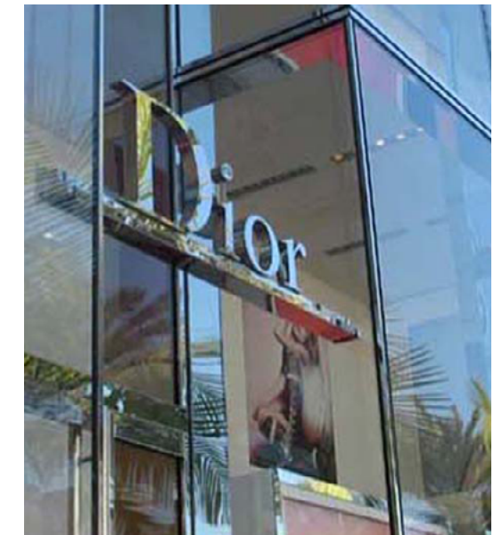
Primary Sign: Signage shelf with hidden uplight and finished letterforms.
