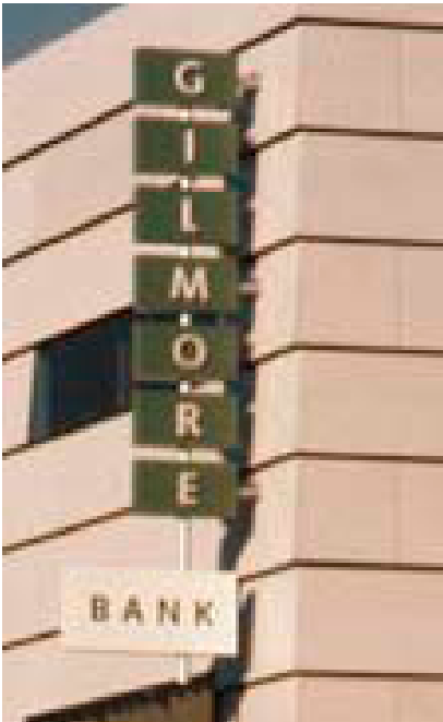
Primary Sign: Combination of open pan channel letterforms with recessed exposed neon and internally illuminated metal face with push-through acrylic letterforms.
