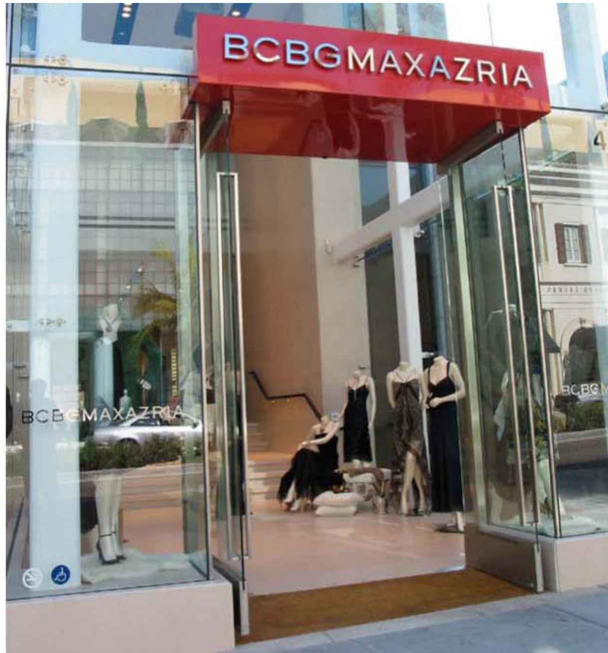
Primary Sign: Metal canopy has reverse channel dimensional halo-lit letterforms.
