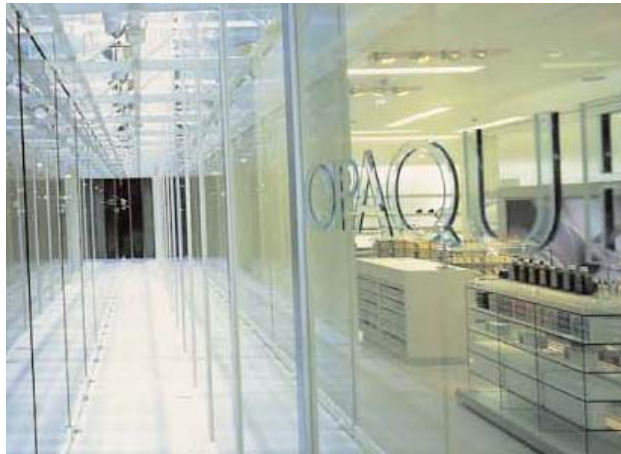
Primary Sign: Clear glass letterforms with polished edges surface mounted to glass panel.
