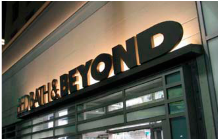
Primary Sign: Reverse channel dimensional halo-lit letterforms.
