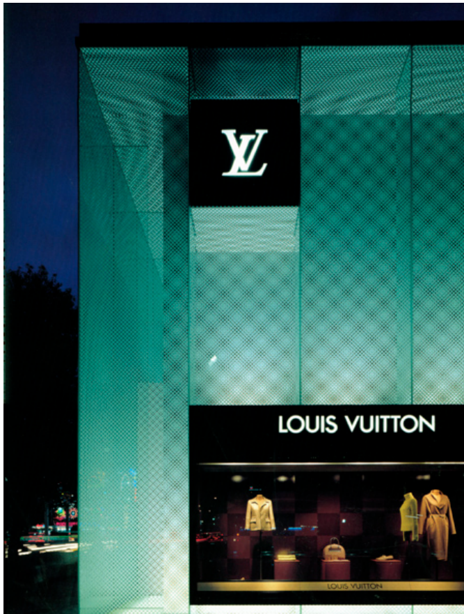
Primary Sign: Internally illuminated metal face with acrylic letter forms. Secondary sign above is same construction.
