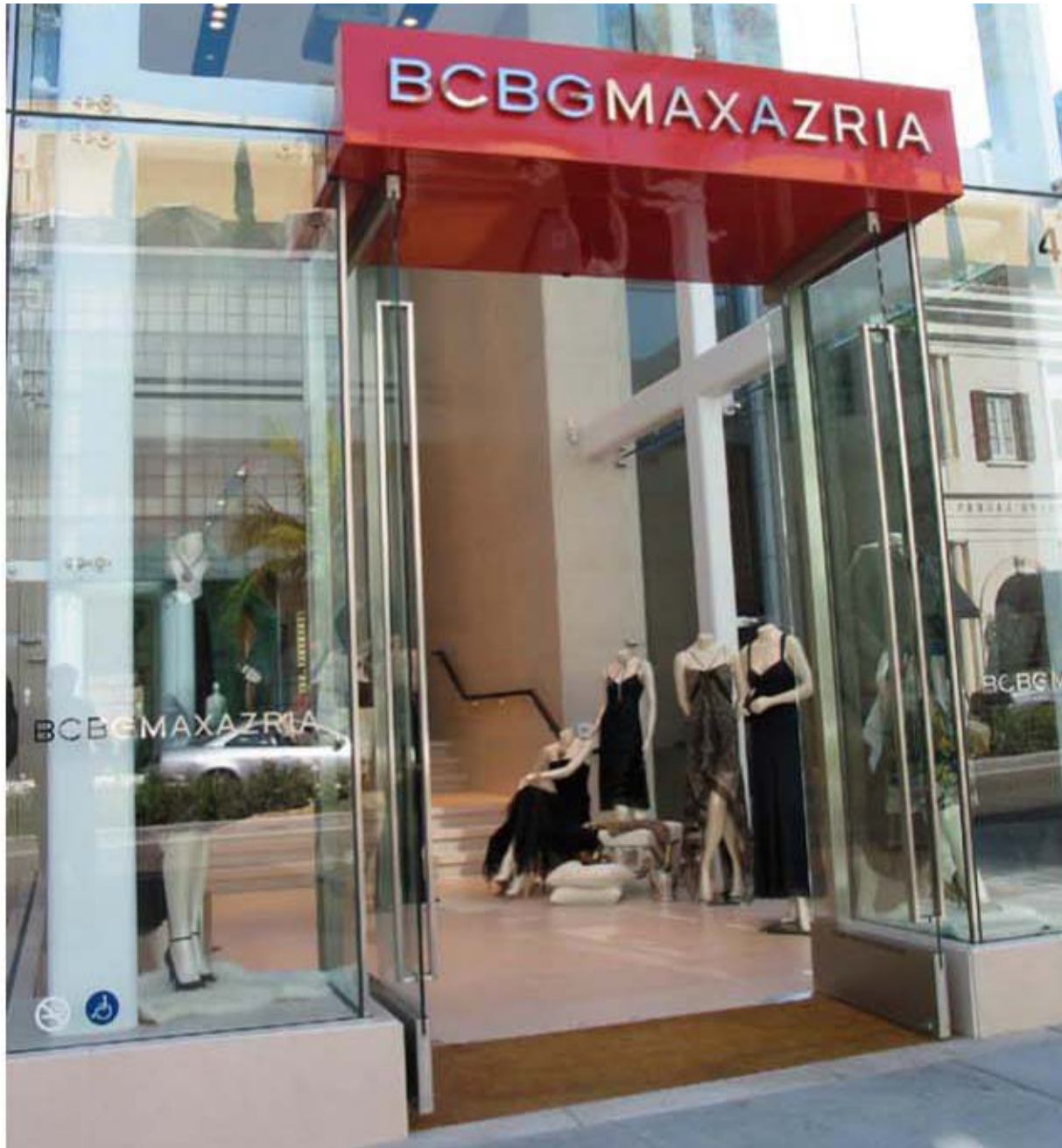
Primary Sign: Metal canopy has reverse channel dimensional halo-lit letterforms.
