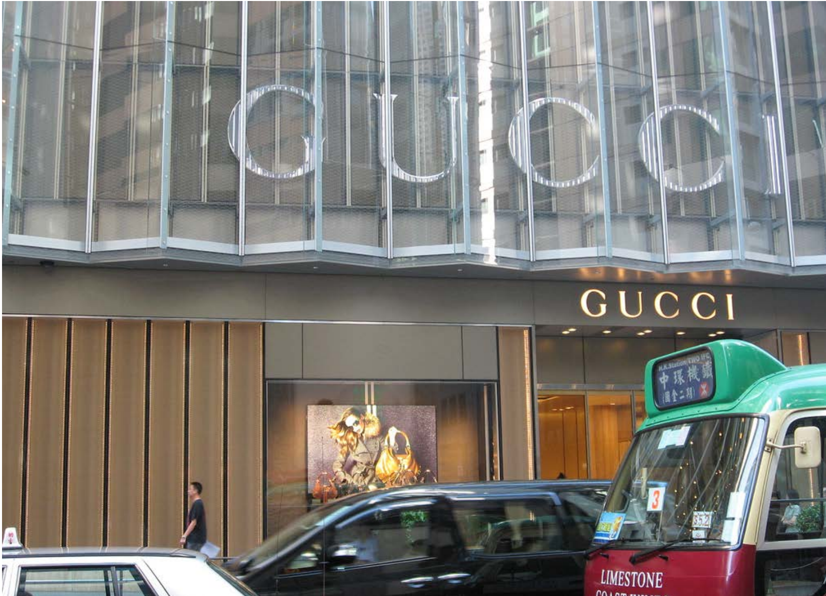
Secondary Sign: Laser cut metal letters are pinned from storefront behind glass.
