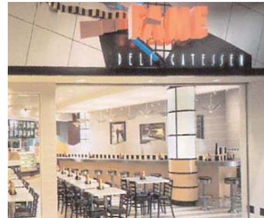
Primary Sign: Combination of reverse channel halo-lit letterforms and internally illuminated metal letterforms with push-through acrylic face.
