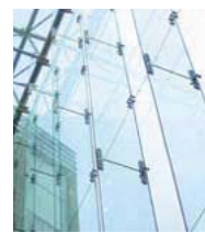
Structural Fin Glass System (Inside View)
