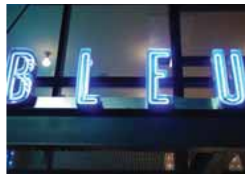
TYPE B. Open pan channel letterforms with recessed exposed neon.
