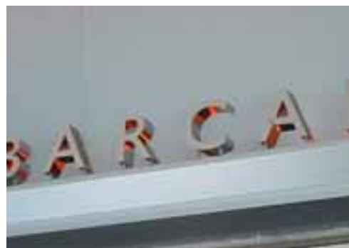
TYPE A. Reverse channel dimensional halo-lit Letterforms mounted to solid background panel
