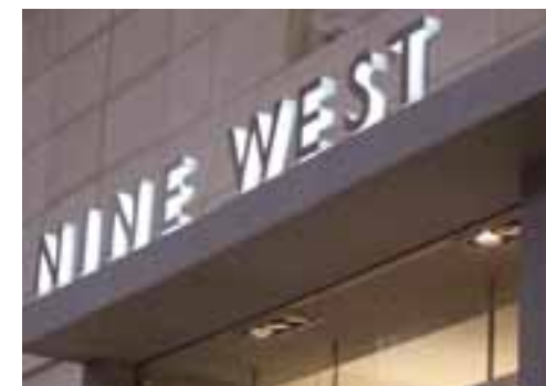
TYPE D. Dimensional graphics or letterforms pinned off solid background panel or attached to a powered signage shelf.
