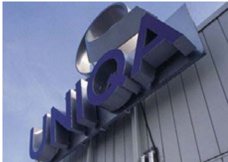
Primary Sign: Halo-lit dimensional letterforms are pinned off panel.
