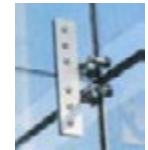
Structural Glass Spider Fitting
