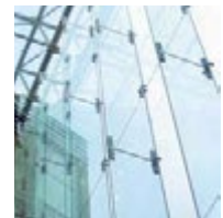
Structural Fin Glass System (Inside View)
