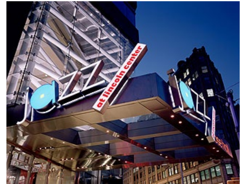
Primary Sign: Individual internally illuminated letterforms with push-through acrylic and halo-lit are pinned off metal canopy.
