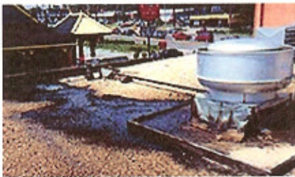
Roof Without Grease Guard Protection
