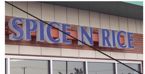
Exposed raceway
