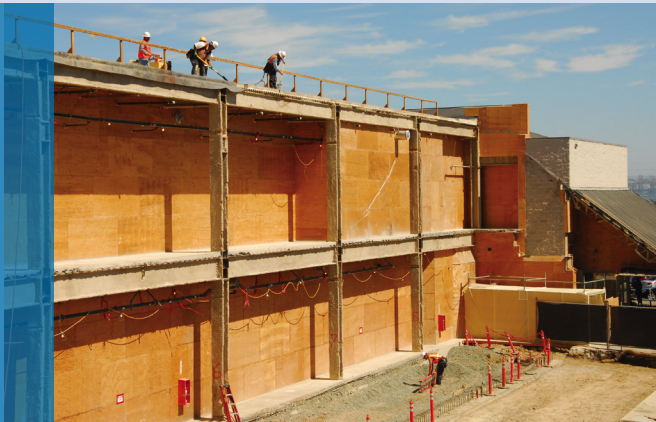
Nordstrom under construction Village at Corte Madera - Corte Madera, CA
